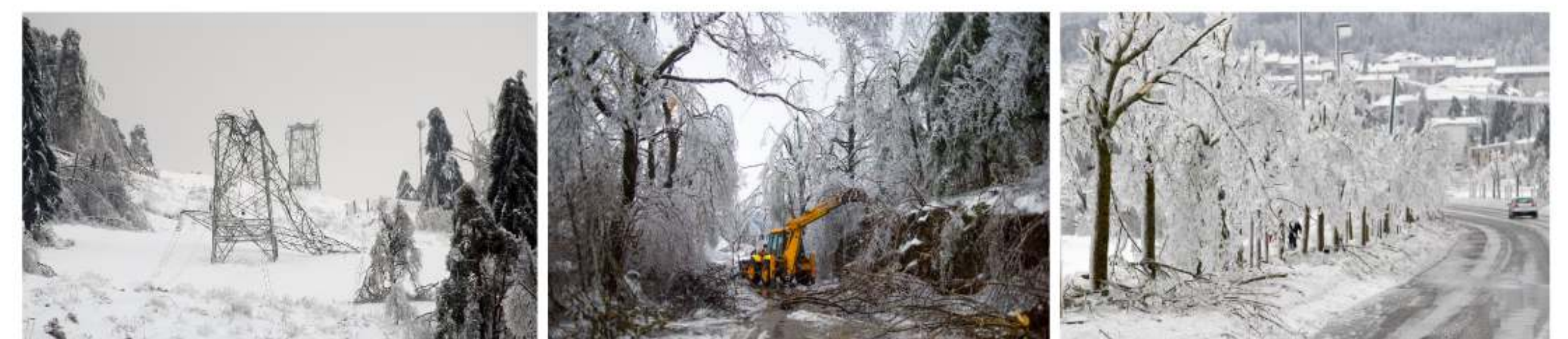
Damage caused by severe freezing rain and ice.
